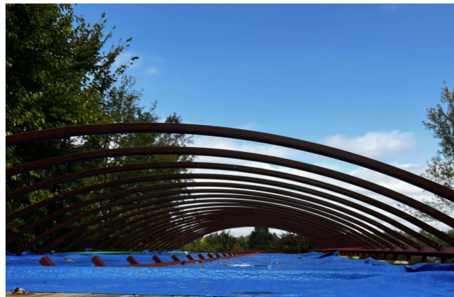
D. Also secure each rib to ridge beam
