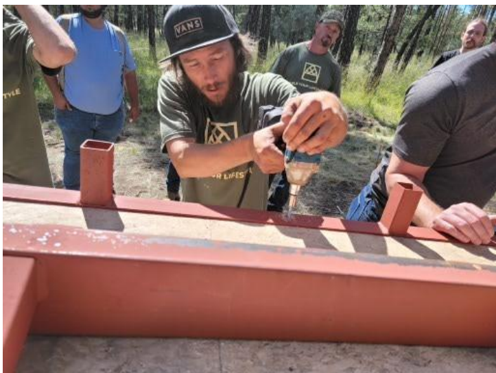
A. Secure the base plate through pre drilled holes
