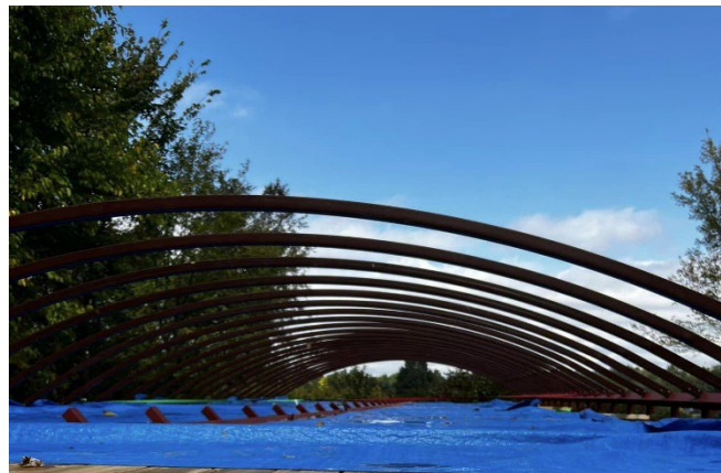
D. Also secure each rib to ridge beam
