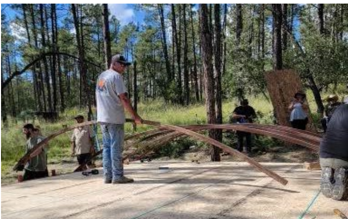
C. Attach each rib to chained plate
